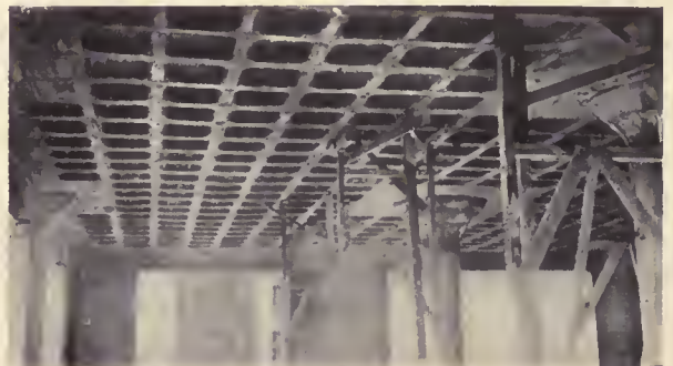
LOOKING UP AT UNDER SIDE OF SLAB Forms have been removed
